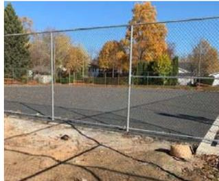
The fencing has just been completed and the asphalt has been laid. The final touch will be the entry gates and the final colour coating which will be applied in the Spring of next year.
